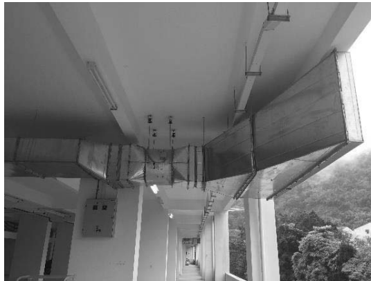
Installation of ventilation fan system for a high rise residential property in Selangor
