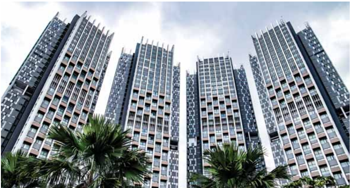
Lumi Tropicana has achieved Green Building Index certification in FY2021.
