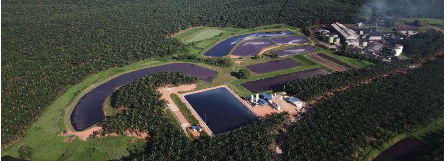
The Cenergi Lawiang 1.2MW Biogas Power Plant in Kluang, Johor.
