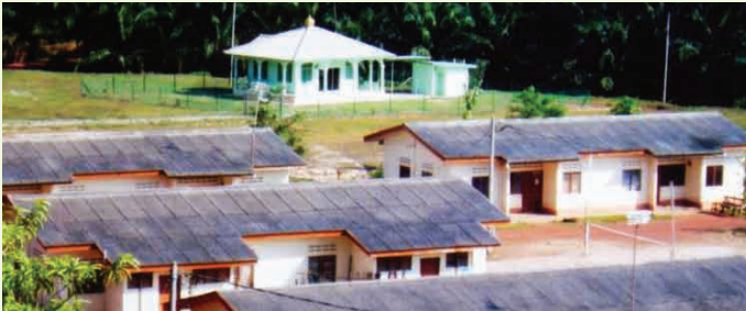
Housing complex provided by THPB for its plantation workers in Kota Bahagia, Pahang.
