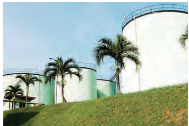
Depot for CPO Storage Tanks at the Kota Bahagia Mill.
