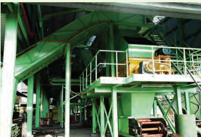
The front-end of the Kota Bahagia Mill which is currently being upgraded from a conventional cage-based conveyor system to that of a continuously sterilised production flow system
