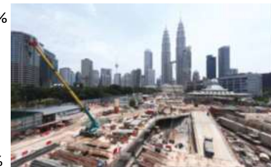
KLCC North East Car Park, Package 2 & 2A
