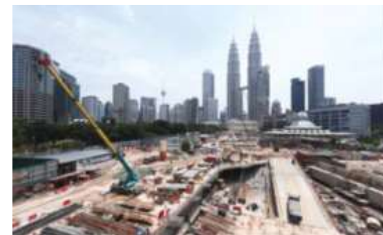
KLCC North East Car Park, Package 2 & 2A
