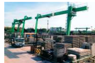
Precast Yard in Singapore
