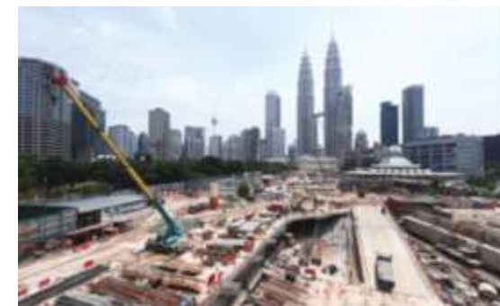
KLCC North East Car Park, Package 2 & 2A
