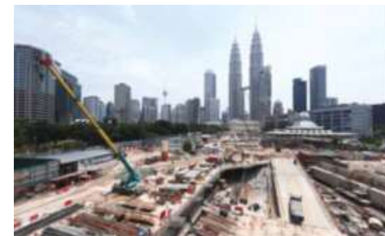
KLCC North East Car Park, Package 2 & 2A
