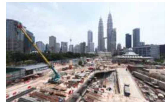
KLCC North East Car Park, Package 2 & 2A
