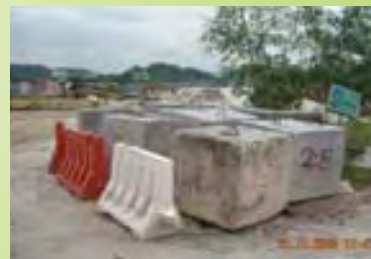
Excess concrete cast as counter-weight
