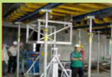
Use of system formwork
