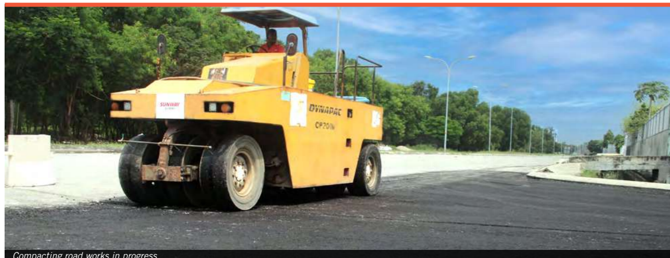
Compacting road works in progress
