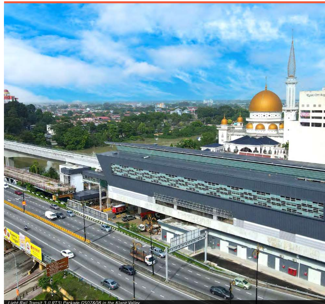
Light Rail Transit 3 (LRT3) Package GS07&08 in the Klang Valley
