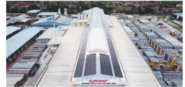
Batang Kali plant rooftop PV solar panels
