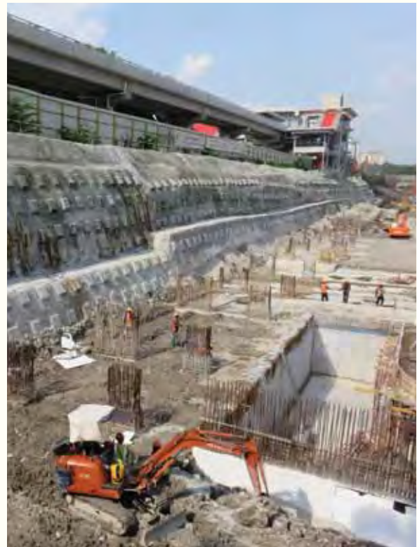
SLOPE STABILISATION FOR SUNWAY GEO COMMERCIAL PRECINCT Bandar Sunway
