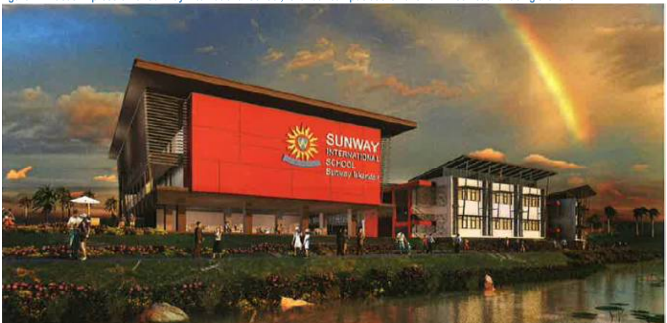
Figure 2: Artist's impression of Sunway International School, Iskandar campus at the Lakeview Precinct and facing the lake
