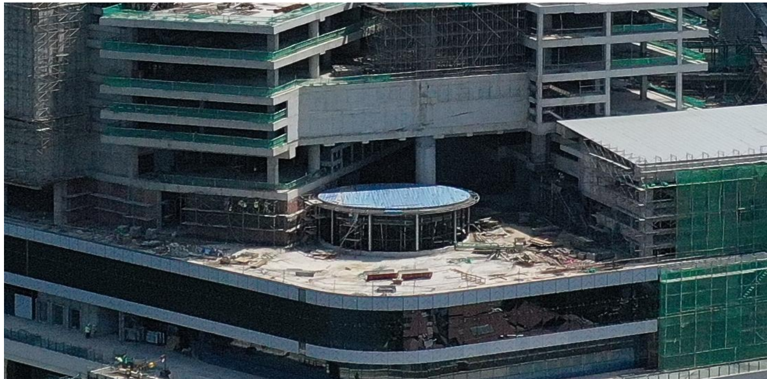
Sunway Square – District Cooling System
