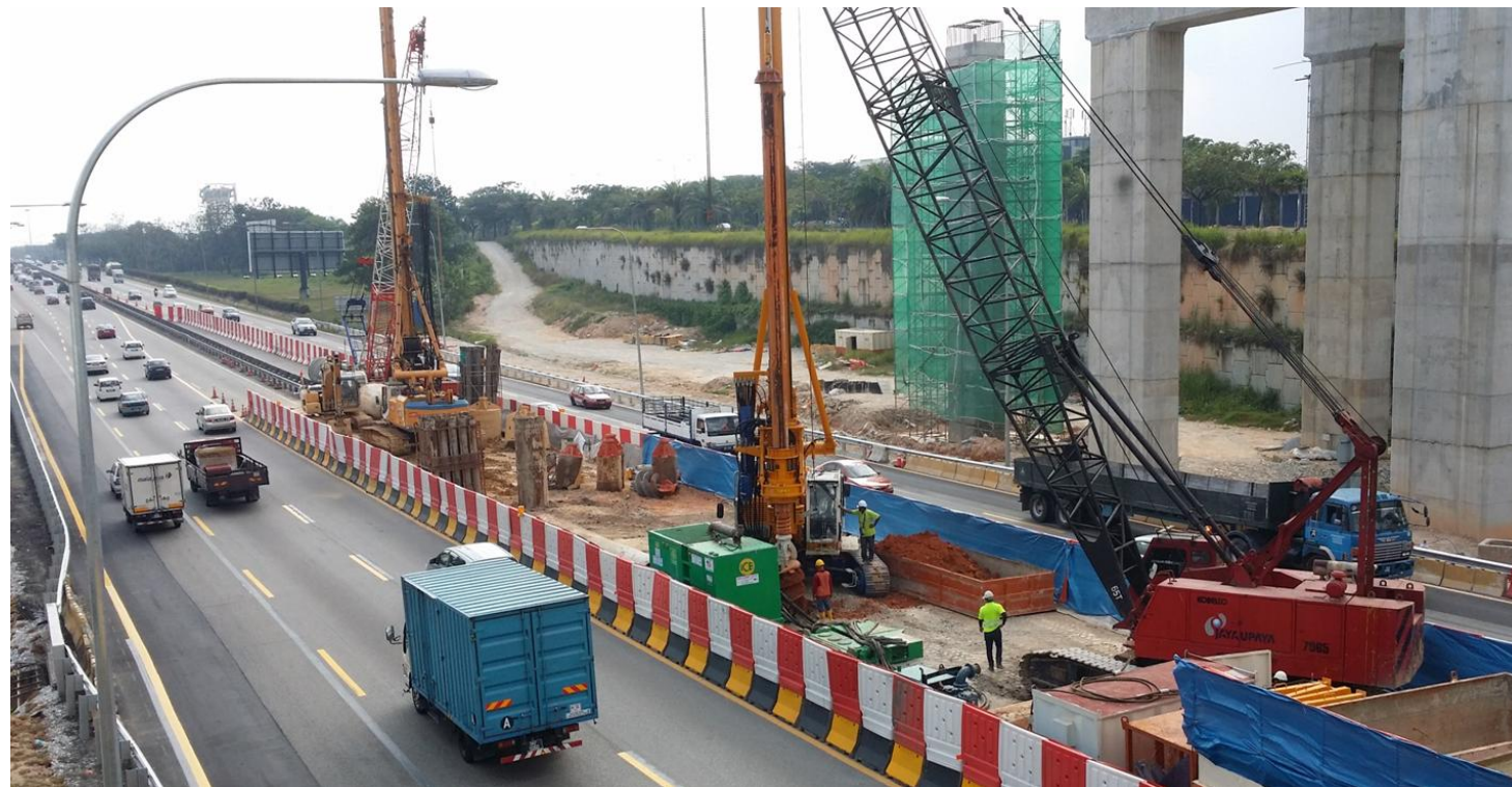
Pile Foundation Works
