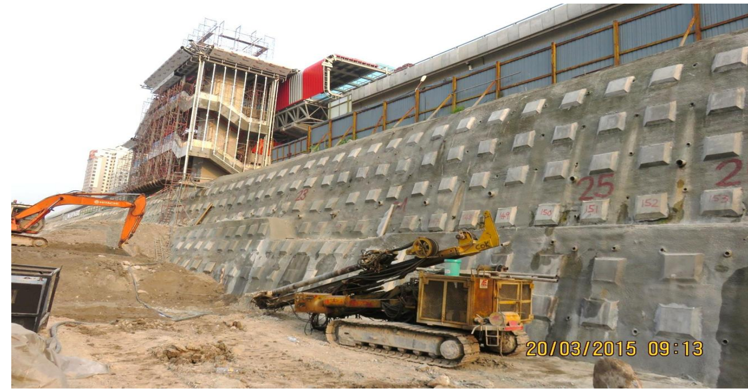
Earth Retaining System
