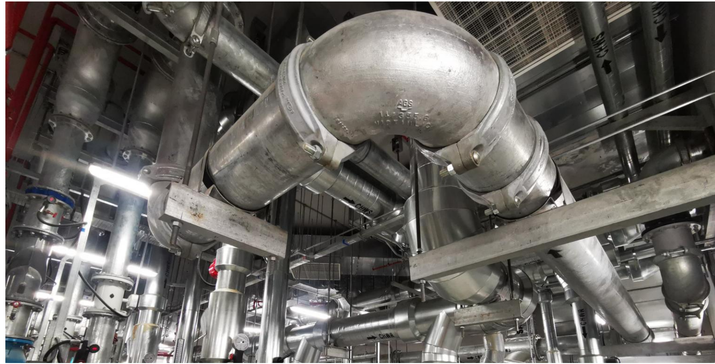
MRT Sentul West Underground Station
