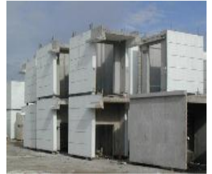
Lift Core Wall
