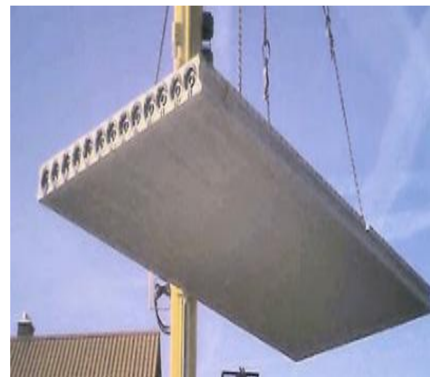
Hollow Core Slab
