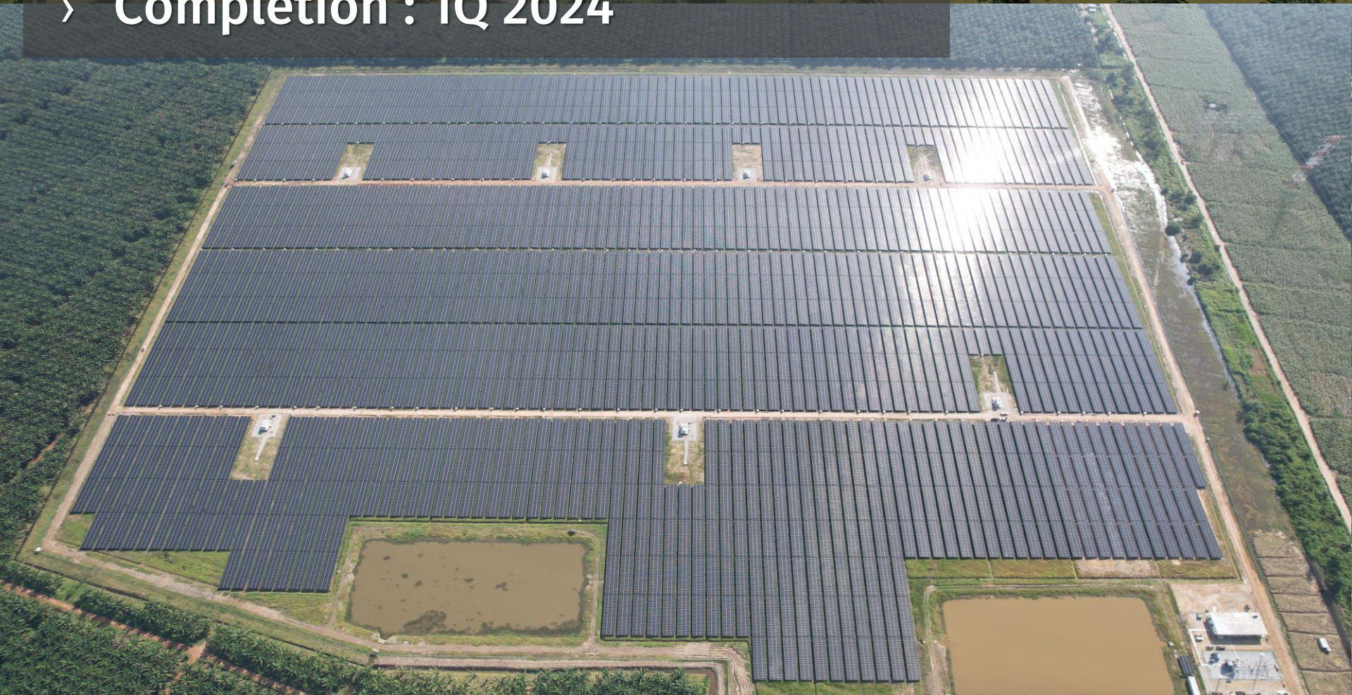
Large Scale Solar 4, Kapar, Klang (50MW)
