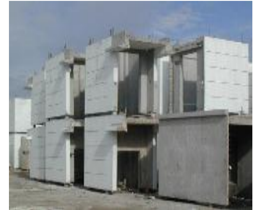
Lift Core Wall
