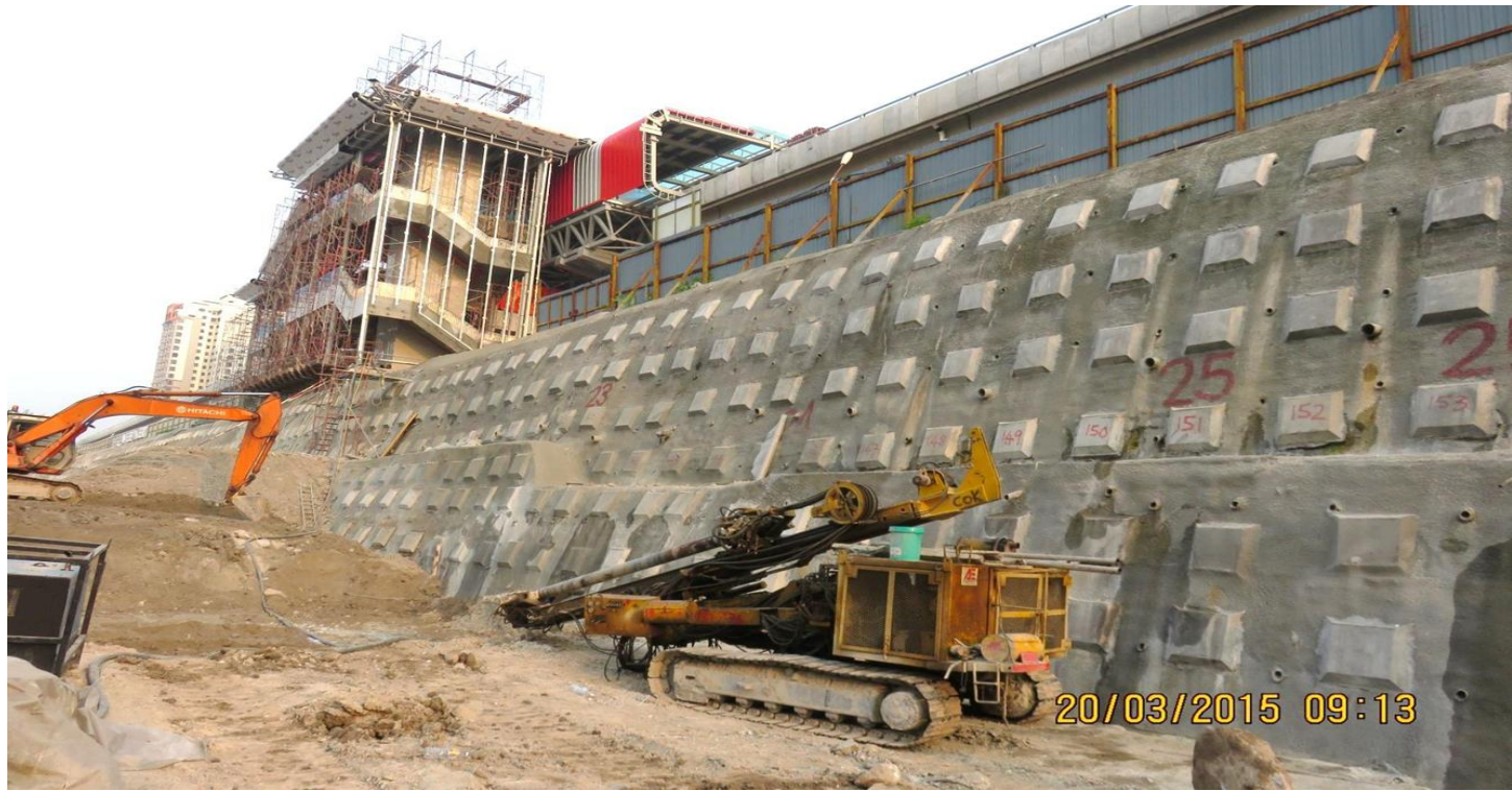
Earth Retaining System
