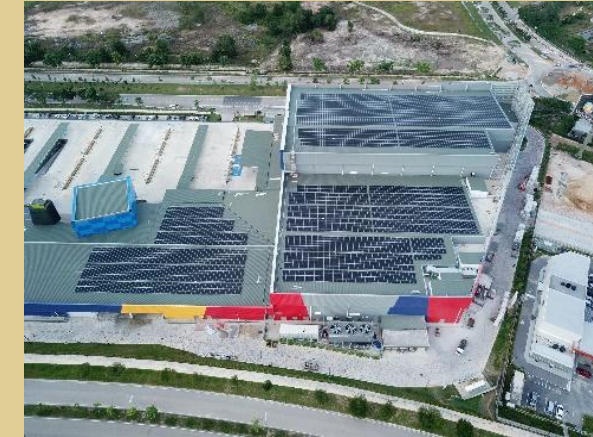
Sustainable Energy Services
