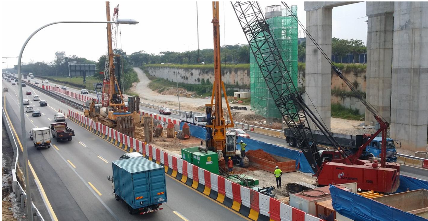
Pile Foundation Works
