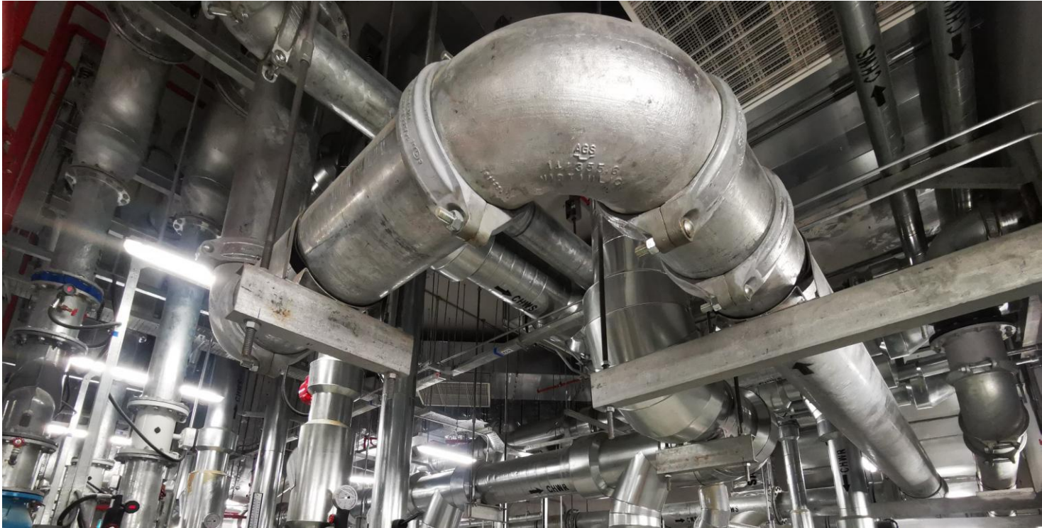
MRT Sentul West Underground Station
