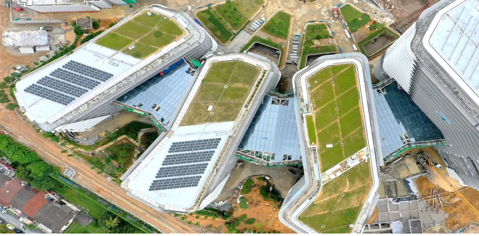
TNB HQ Campus Phase 2 – KL
