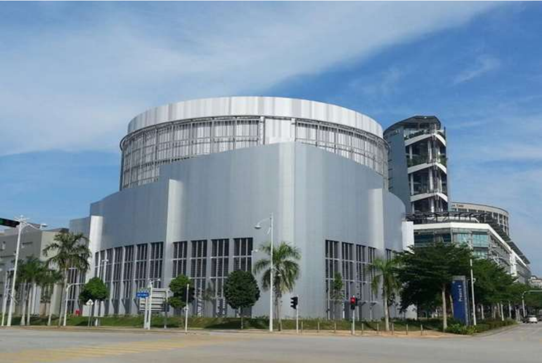
Gas District Cooling Plant - Putrajaya
