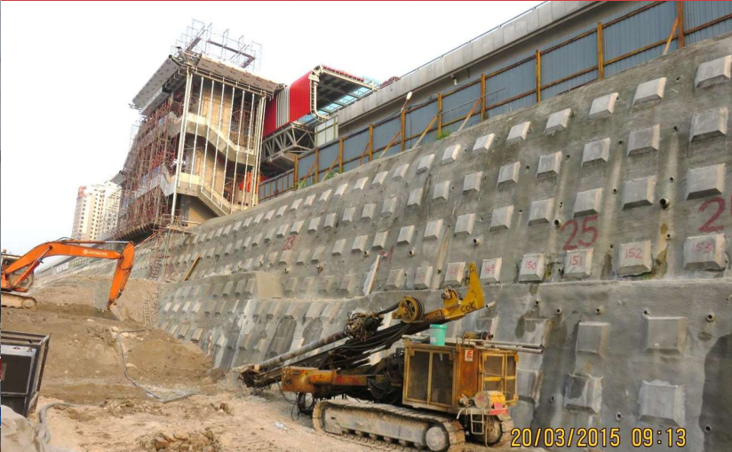
Earth Retaining System
