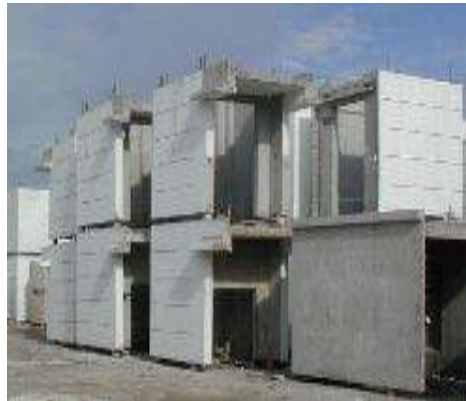
Lift Core Wall
