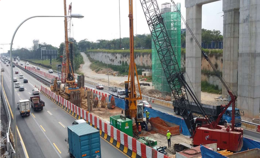
Pile Foundation Works
