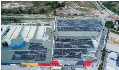
Sustainable Energy Services
