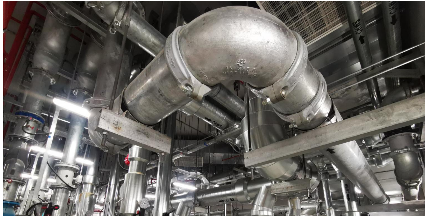
MRT Sentul West Underground Station
