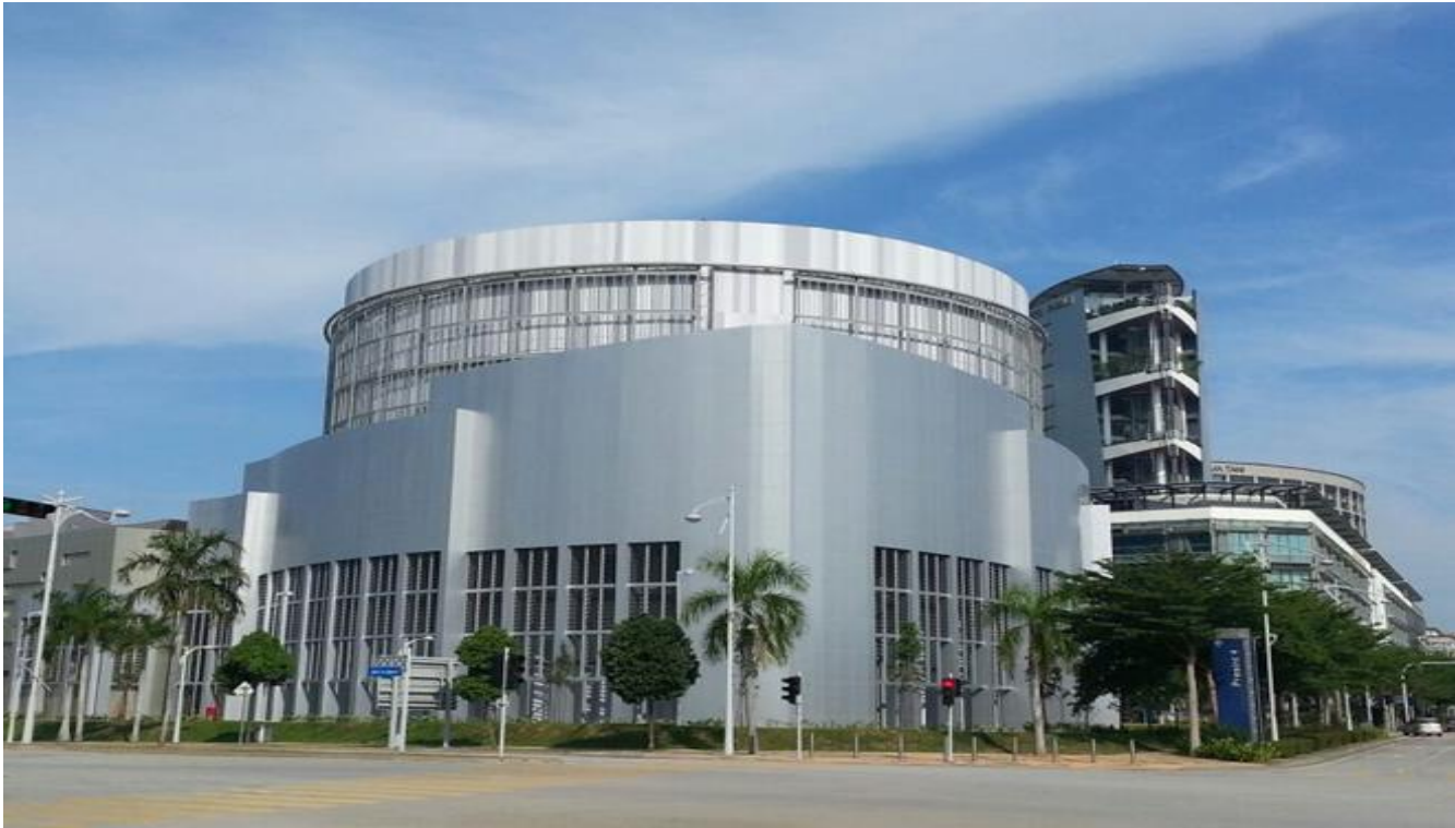
Gas District Cooling Plant - Putrajaya
