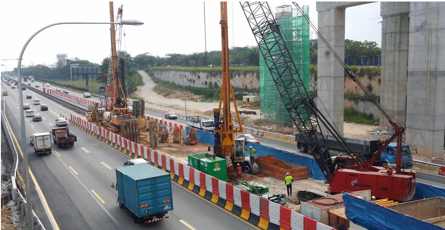
Pile Foundation Works
