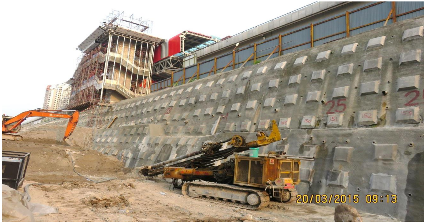
Earth Retaining System
