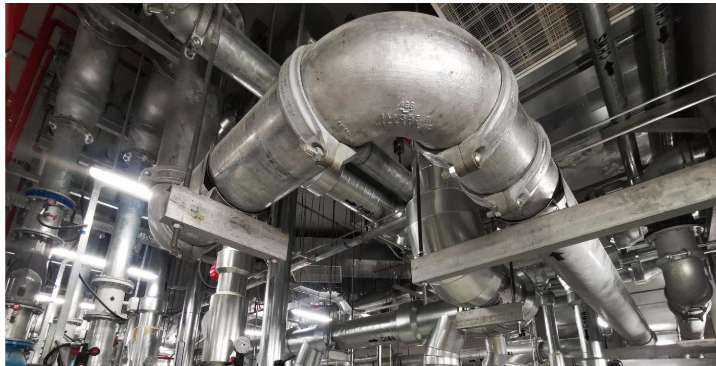
MRT Sentul West Underground Station
