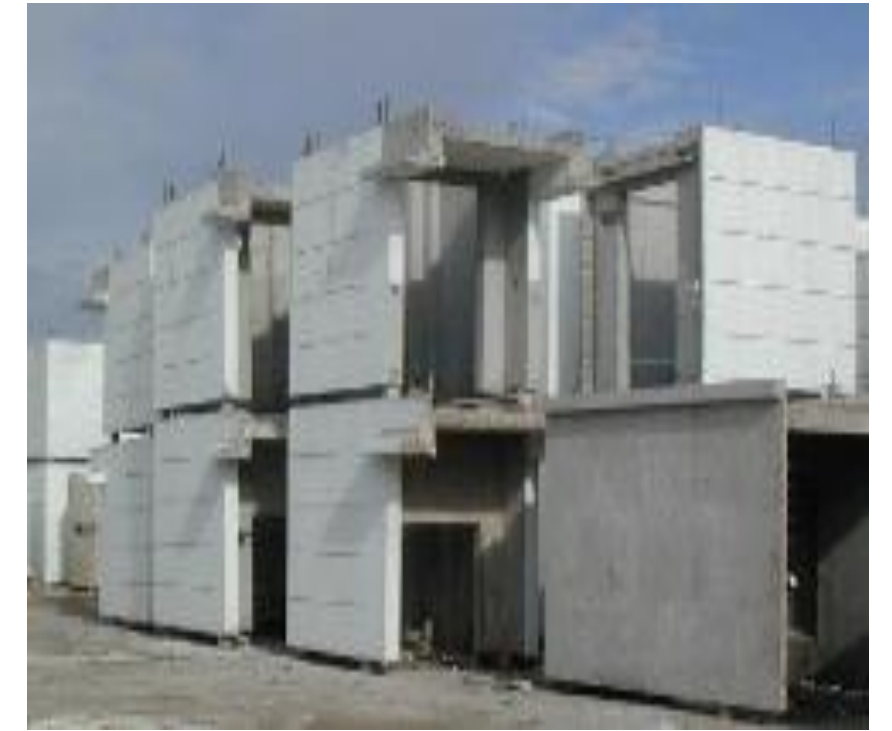
Lift Core Wall
