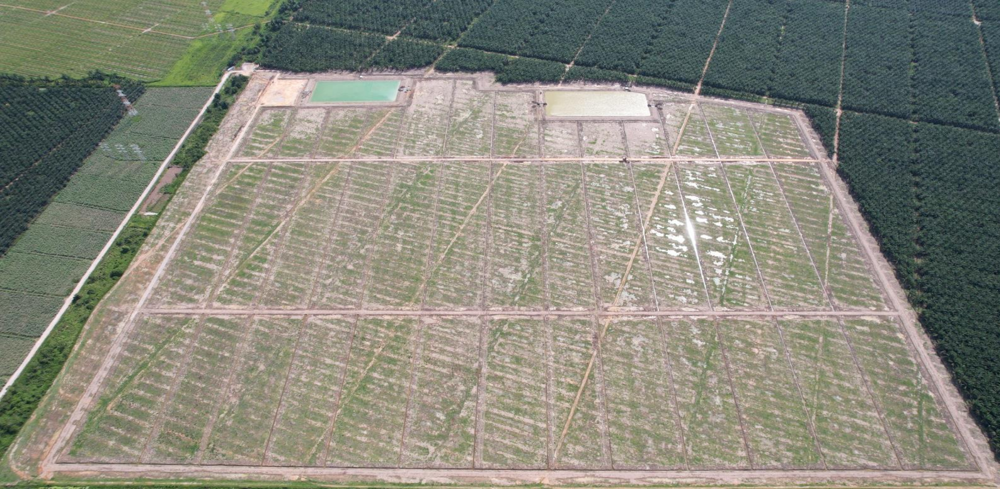
Large Scale Solar 4, Kapar, Klang (50MW)
