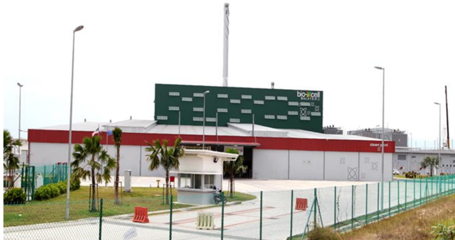
Central Utilities Facilities
