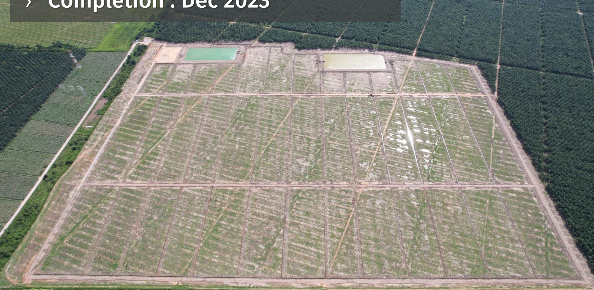
Large Scale Solar 4, Kapar, Klang (50MW)
