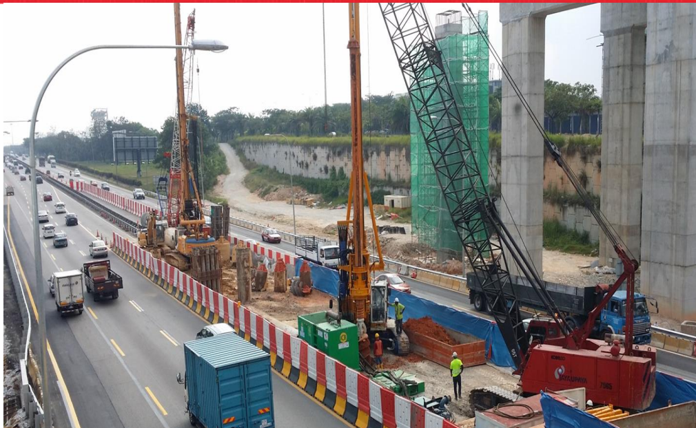
Pile Foundation Works
