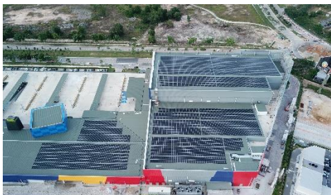
Sustainable Energy Services
