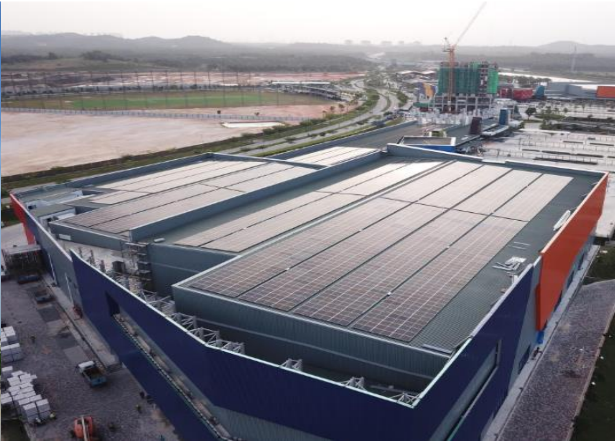
Roof Top Solar – Sunway Iskandar
