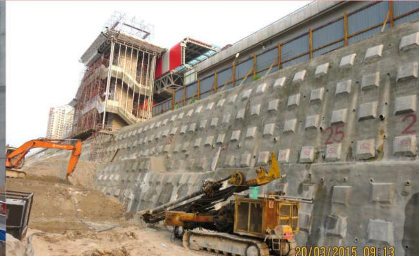
Earth Retaining System
