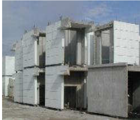
Lift Core Wall
