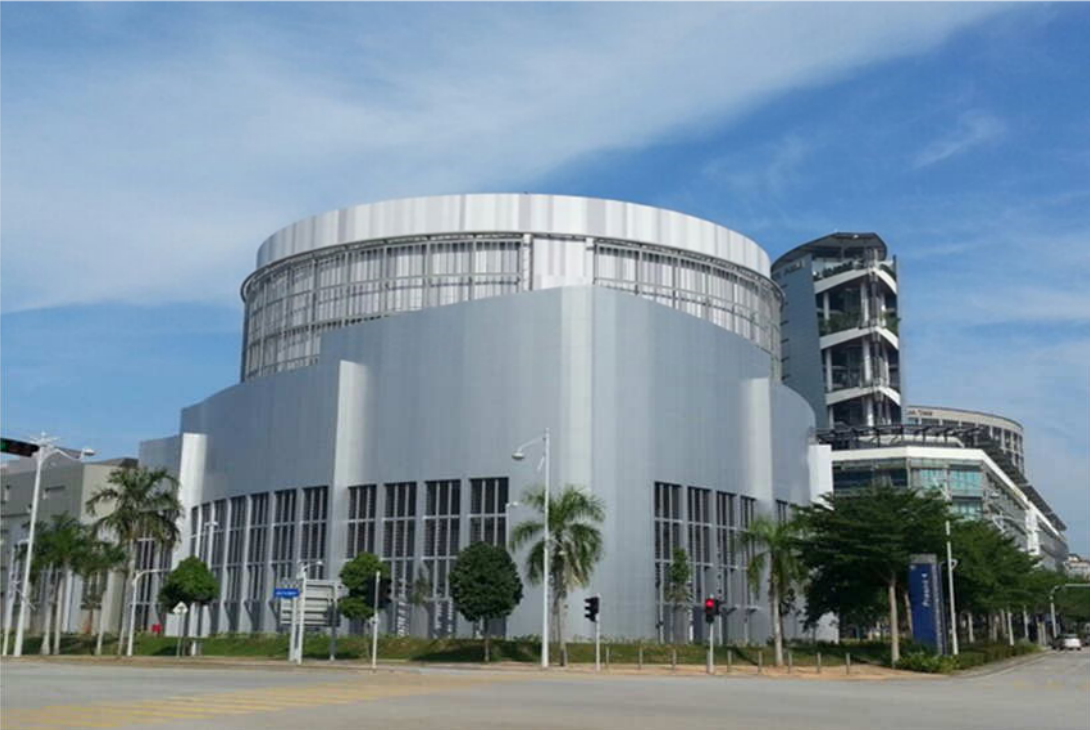
Gas District Cooling Plant - Putrajaya
