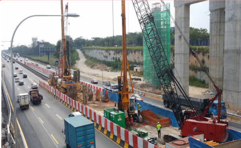
Pile Foundation Works
