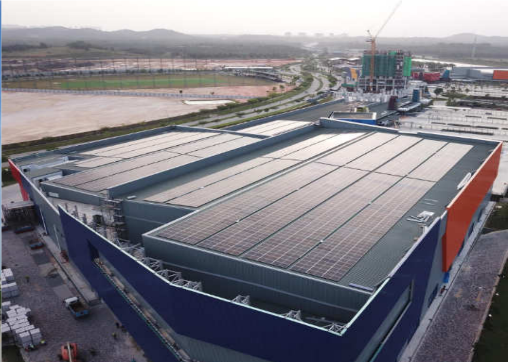
Roof Top Solar – Sunway Iskandar
