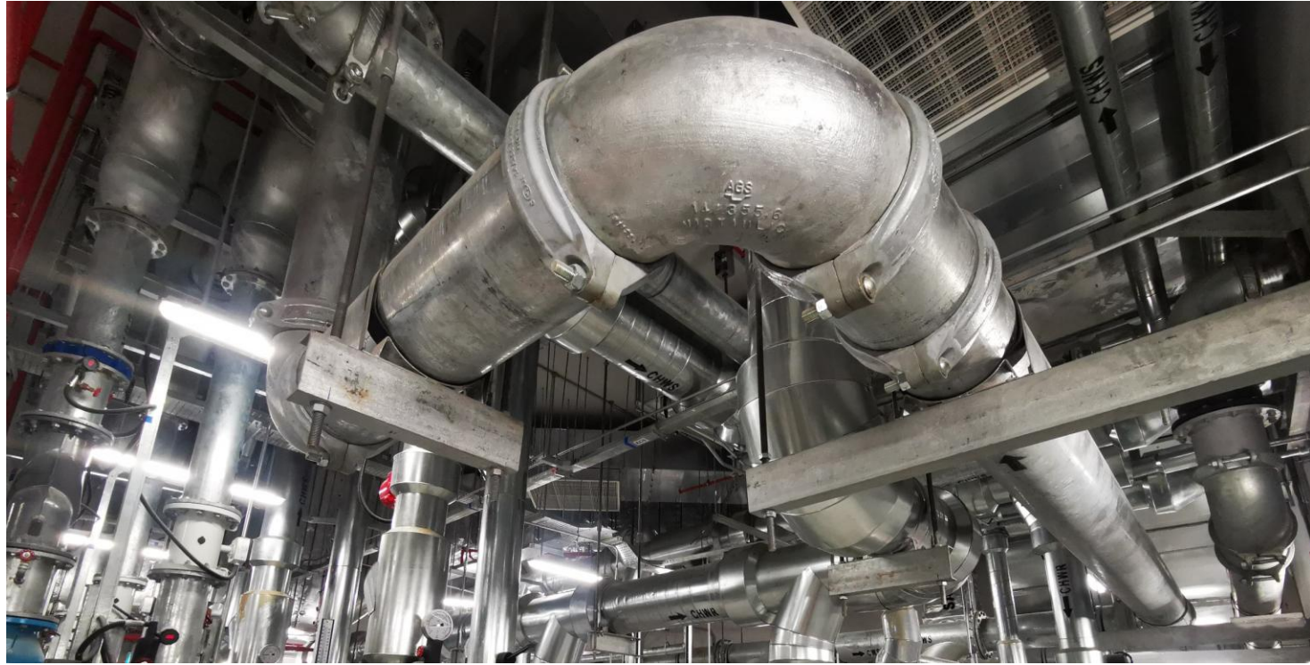
MRT Sentul West Underground Station
