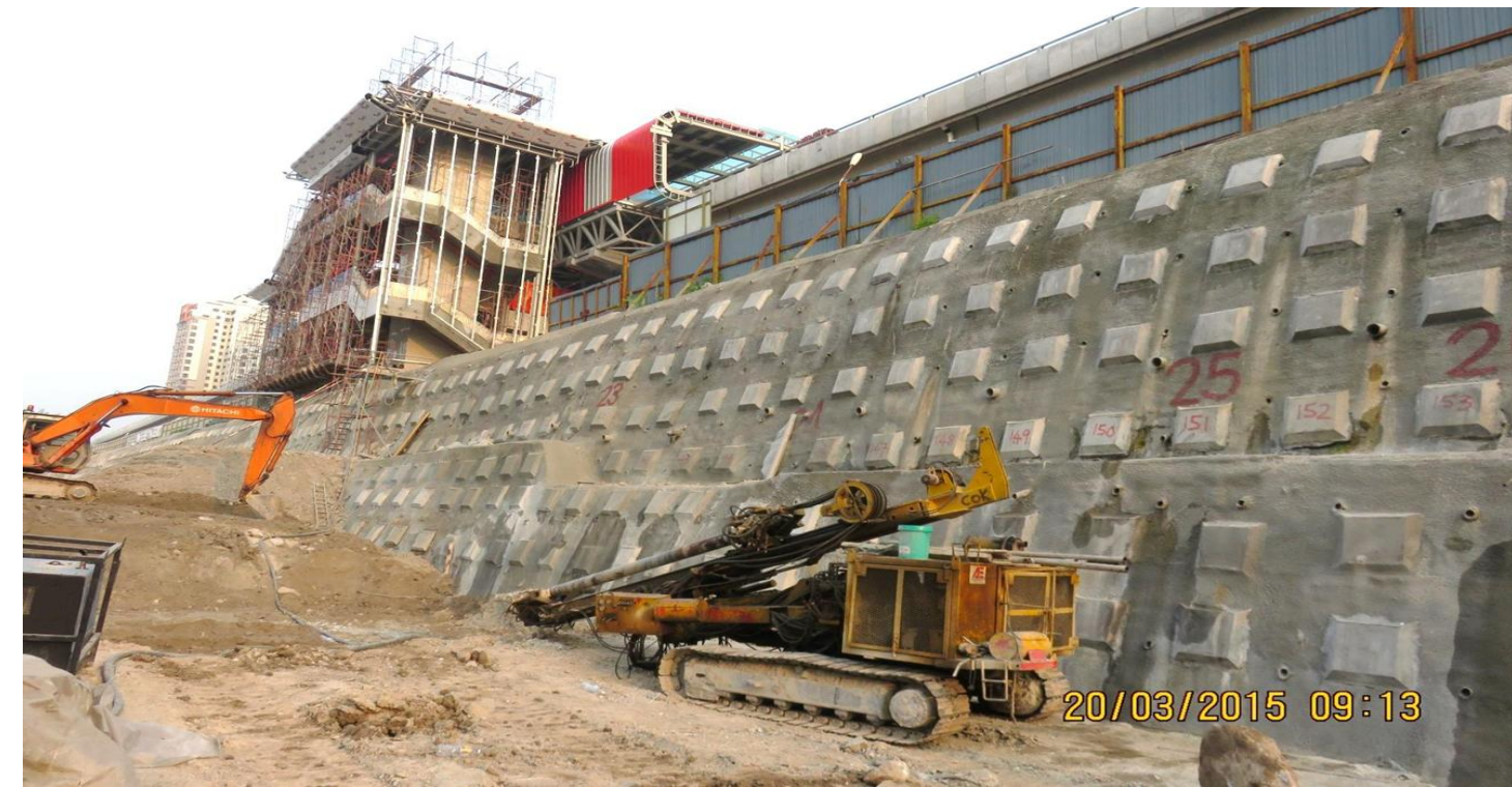
Earth Retaining System
