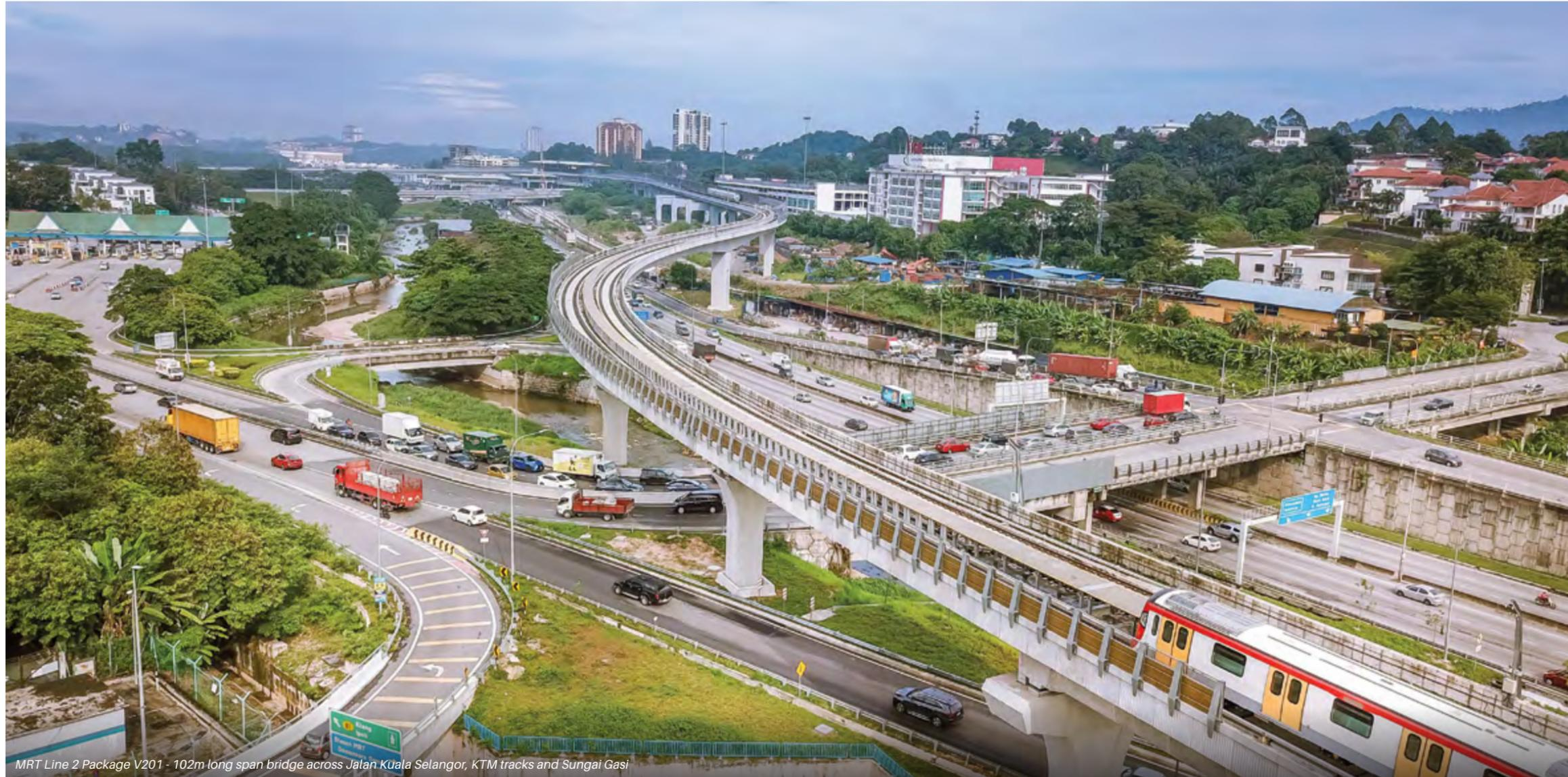
MRT Line 2 Package V201 - 102m long span bridge across Jalan Kuala Selangor, KTM tracks and Sungai Gasi
