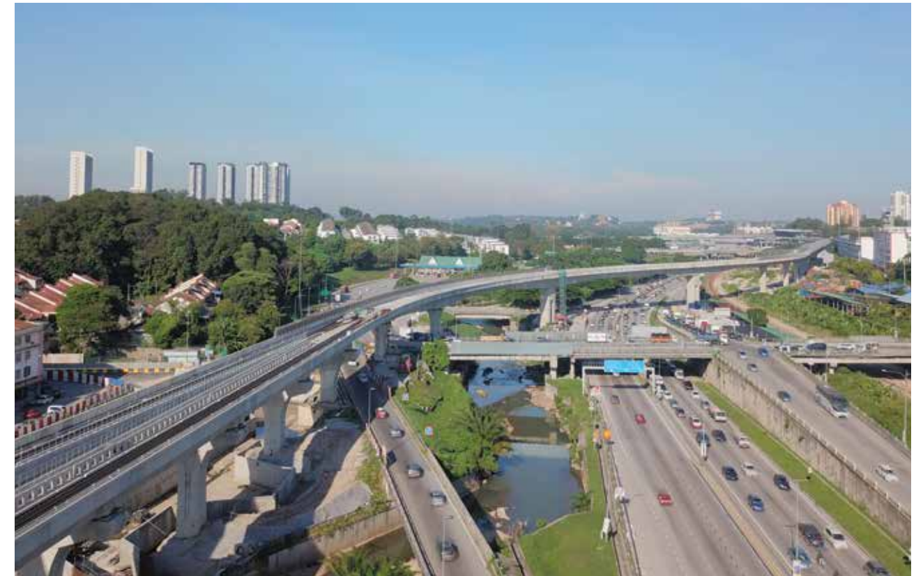
MRT Line 2 Package V201 - 102m long span bridge across Jalan Kuala Selangor, KTM tracks and Sungai Gasi
