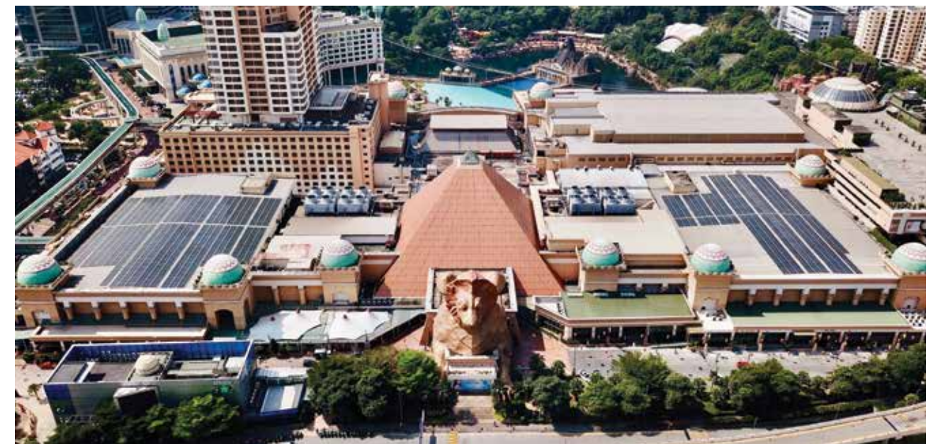
Sunway Pyramid Shopping Centre equipped with solar photovoltaic panels
