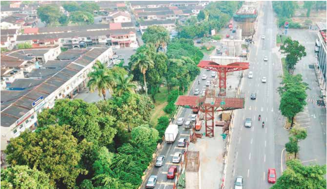
Pier cap works in progress at LRT3 Package GS07&08
