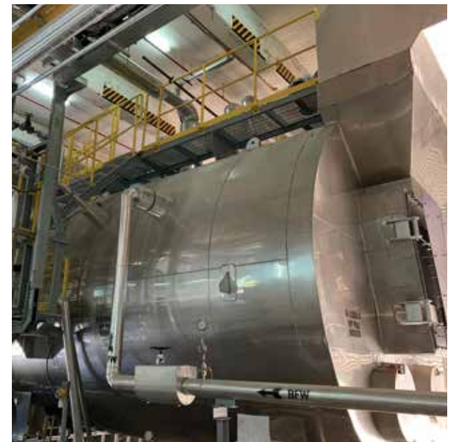
Installation of Auxiliary Gas Boiler and Chilled Water Pump System
