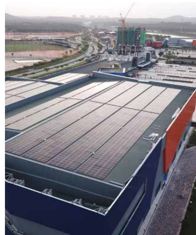
Sunway Big Box Retail equipped with solar photovoltaic panels
