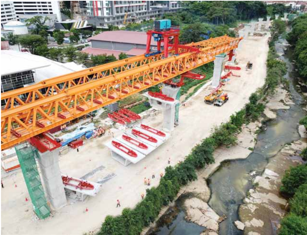
Launching Works at Sri Damansara (MRTV201 Project)
