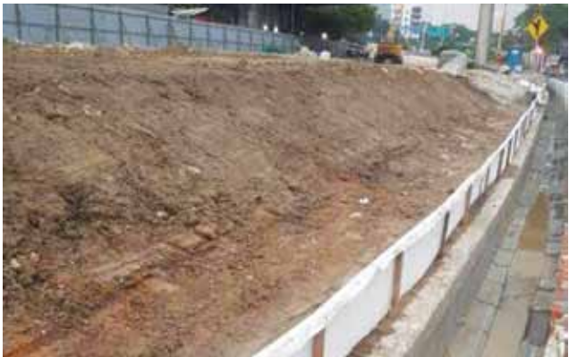
Silt Fence Installed As A Sediment and Erosion Control Measure
