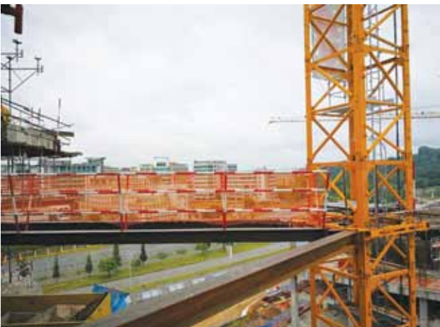
Fall Prevention Measures For Tower Crane Operators
