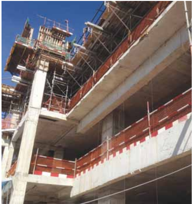
Edge Barricade As A Fall Prevention Measure
