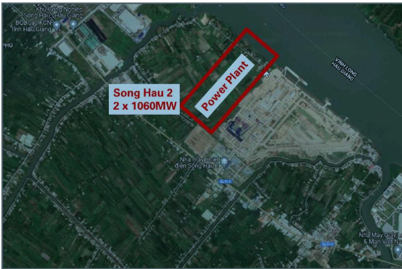
Fig 1: Song Hau 2 Thermal Power Plant project, located at Song Hau Power Generation Centre, Hau Giang Province, Vietnam
