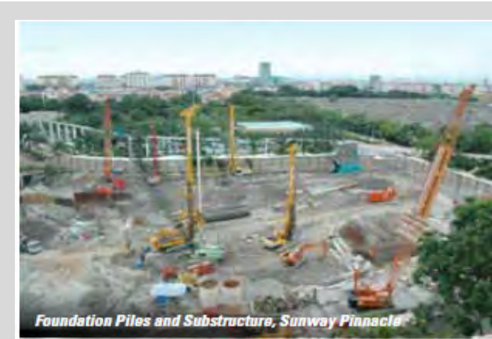
Figure 5: Foundation Piles and Substructure
