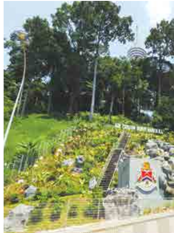
The rehabilitated slopes and waterfall at Bukit Nanas, Kuala Lumpur by Ikram
