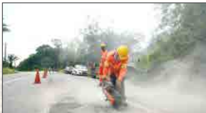
Pavement repair works in progress
