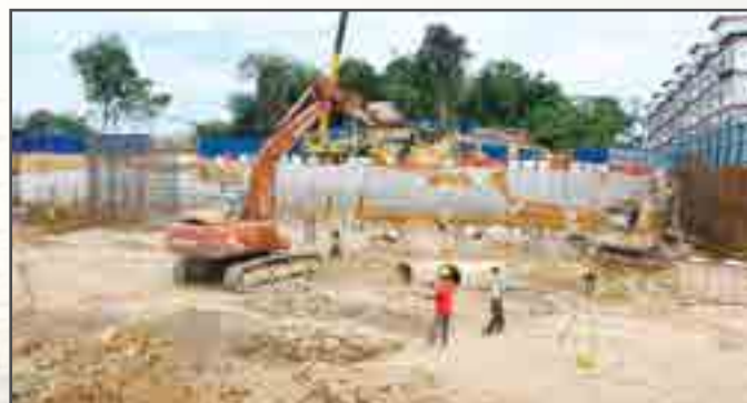
Asian Football Confederation (AFC) Building Project Site
