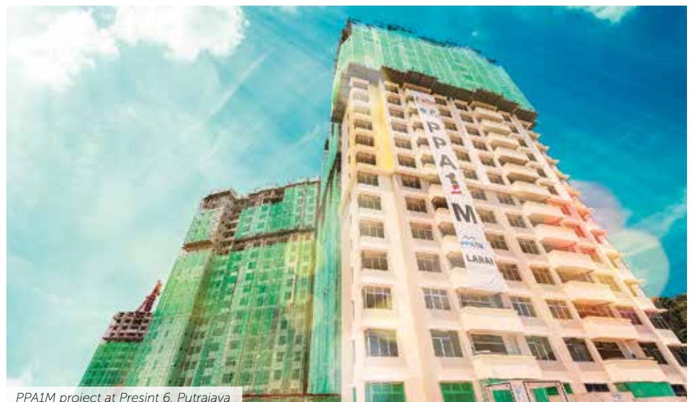
PPA1M project at Presint 6, Putrajaya
