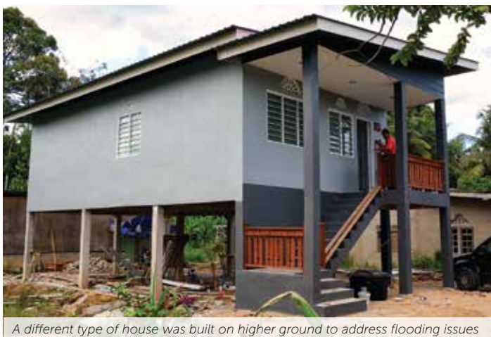
A different type of house was built on higher ground to address flooding issues
