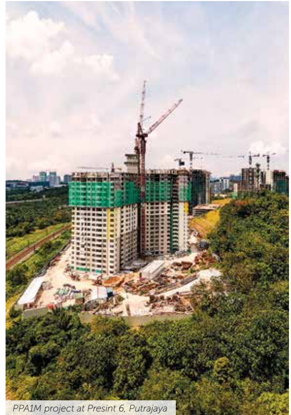
PPA1M project at Presint 6, Putrajaya
