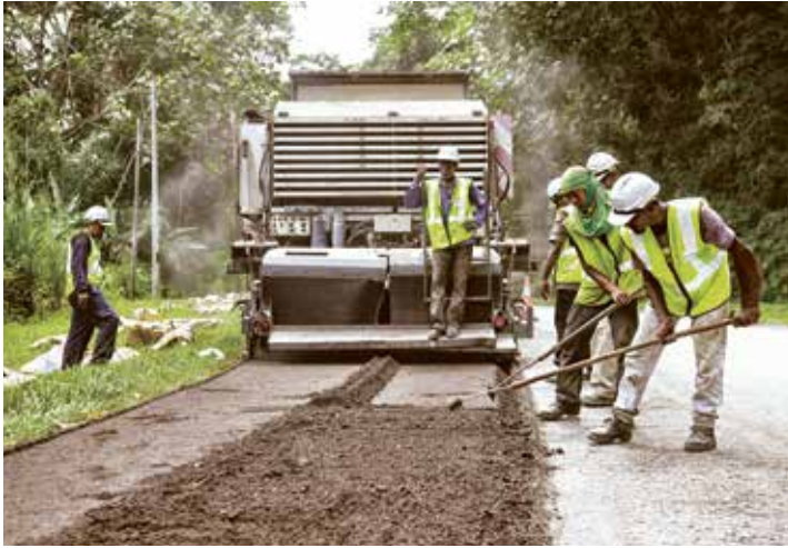
Road maintenance works in Bentong, Pahang
