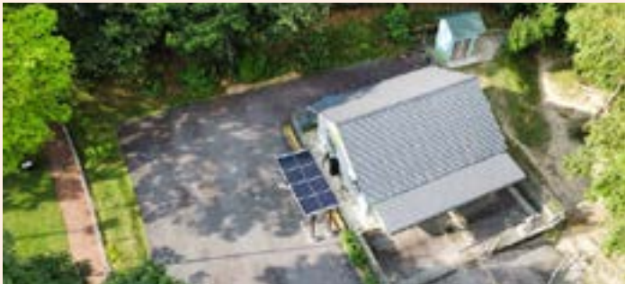
▲ 2.2kWp solar PV system at Kota Damansara Community Forest
