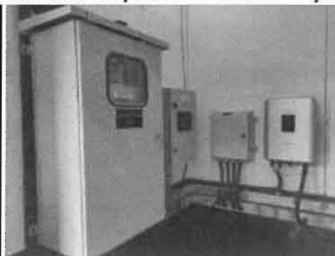
Our energy management system installed as part of a solar PV facility
