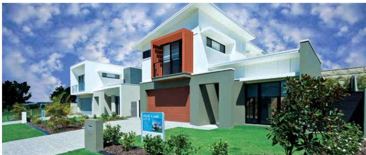
Alpinia, Sanctuary Cove, Australia
