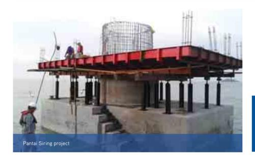
First ever project in Malaysia to install high voltage overhead electricity transmission line crossing over the Strait of Melaka from Pantai Siring to Pulau Besar in Melaka.
