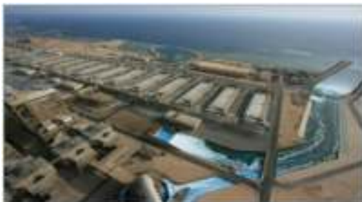
Shuaibah Phase 3 IWPP, Saudi Arabia 105,600 m 3 /day, 108MW
