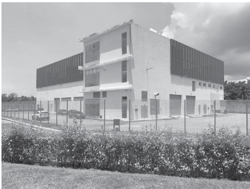
A district cooling plant
