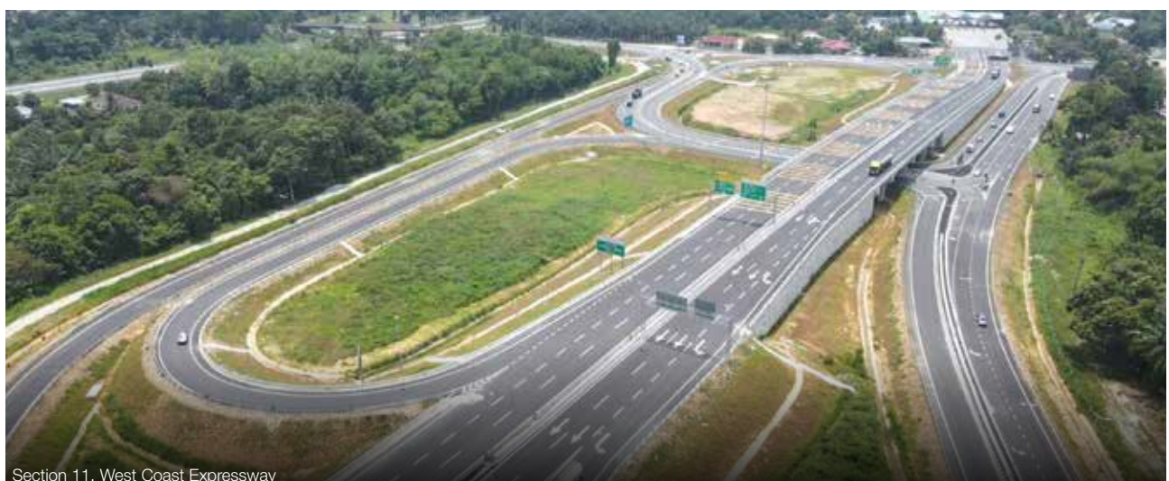
Section 11, West Coast Expressway
