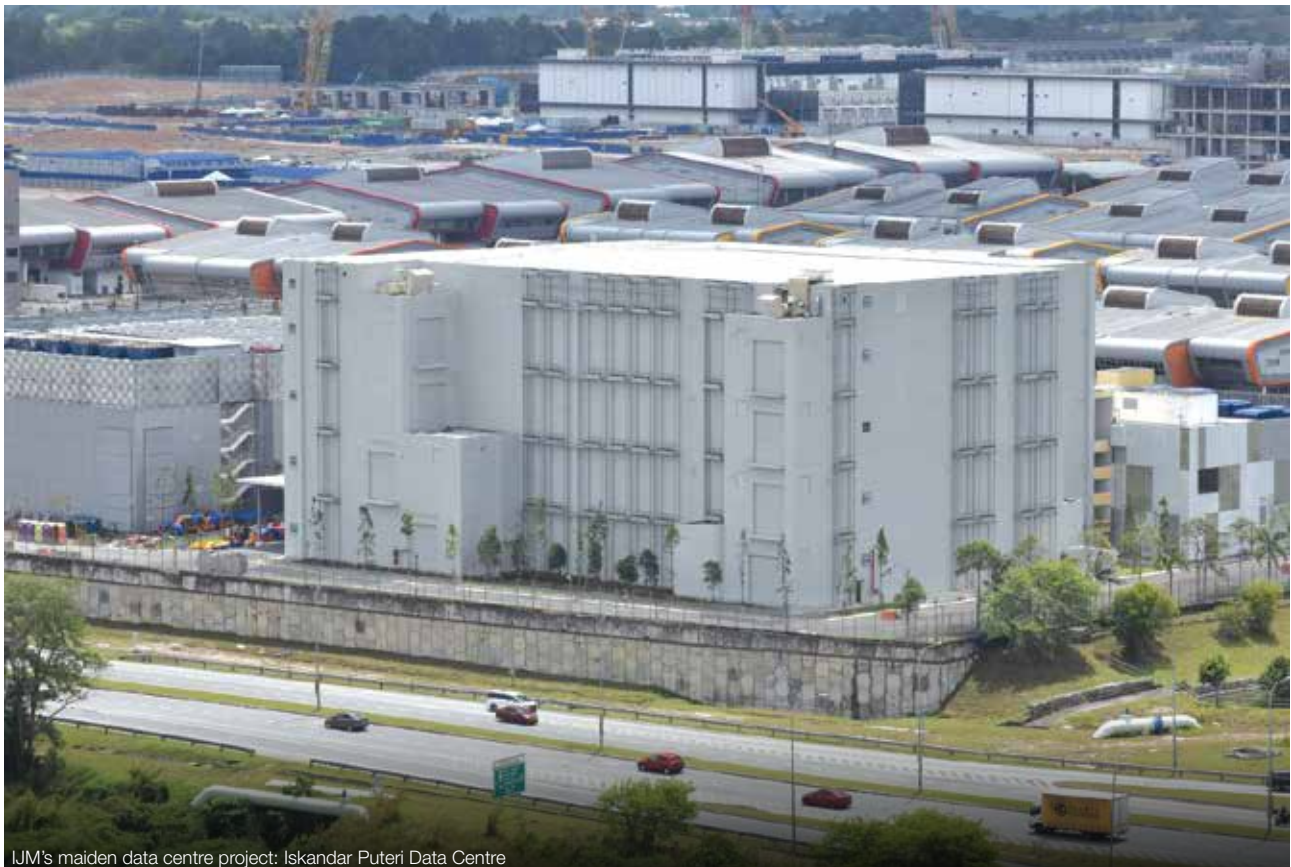
IJM's maiden data centre project: Iskandar Puteri Data Centre
