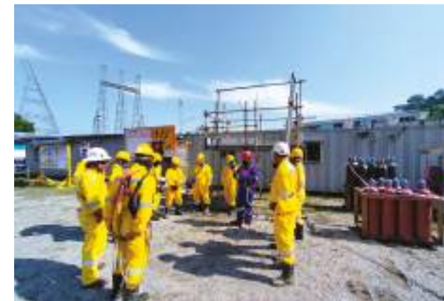
Working At Height (WAH) awareness briefing conducted on 26 May 2023 at a contractor yard.
