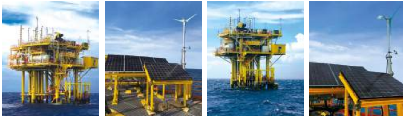
Wind Turbine Solar Hybrid Installation at SFJT-F (2 units).
