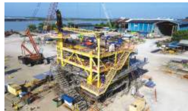
Refurbishment of Topside Platform.
