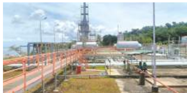
One of the furnaces at LCOT.
