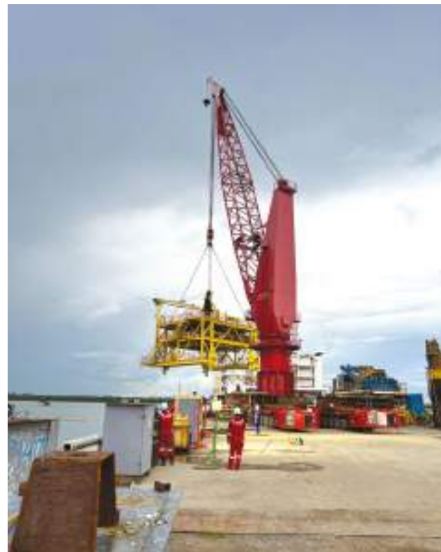
Refurbishment of Topside Platform.
