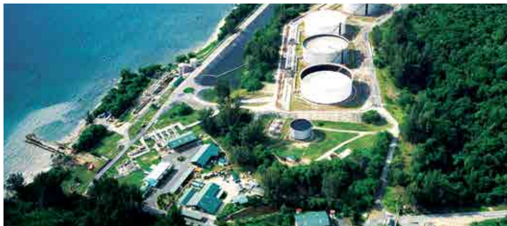
Labuan Crude Oil Terminal (LCOT)
