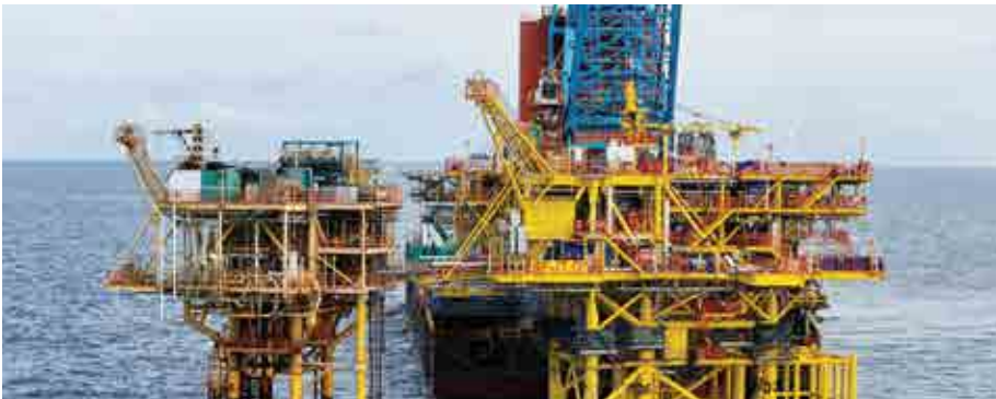
SF30 - New Wellhead Platform as part of SF30 Water Injection Project
