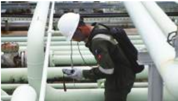
LDAR being conducted at LCOT in December 2022.
