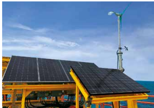
The newly installed solar PV and wind turbine hybrid power at SFJT-F from a different view distance.
