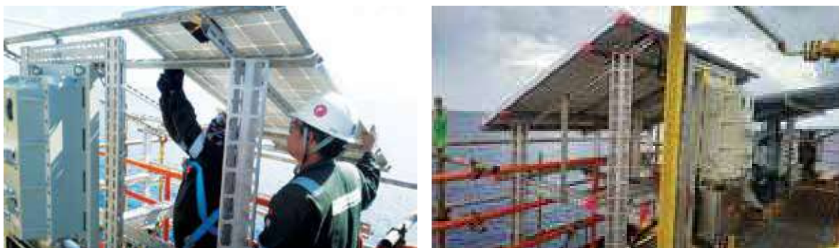
New solar PV system using Hilti Mechano mounting structure in St Joseph SJJT-A – completed in April 2021. Load for well instrumentation.
