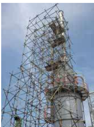
Scaffolding erected at furnace F104 once a year to carry out Dust Particulate monitoring and FBE efficiency assesment.
