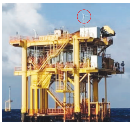
Second wind turbine installed at Barton BTJT-A in late December 2019
