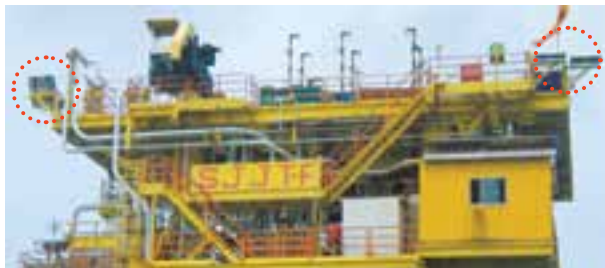
Solar Panel Installation in Saint Joseph Jacket F (SFJT-F) in Malaysia.
