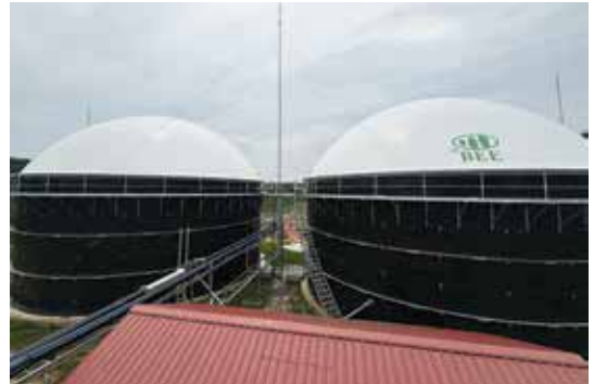
Completed project in FY2025 in Negeri Sembilan, Malaysia
