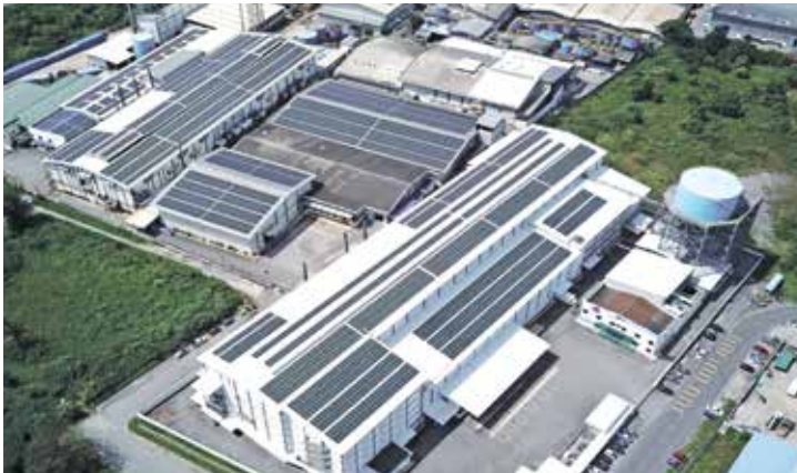
Solar panels installed at Hextar's glove production plants in Ipoh, Malaysia
