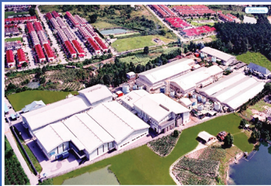
Factory premises in Ipoh, Perak, Malaysia
