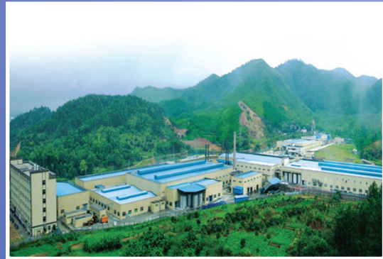
Factory premises in Boluo County, Huizhou City, Guangdong Province, China
